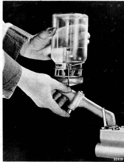
Fig. 38—Filling Brake Master Cylinder with Automatic Refiller (Tool C-362)
